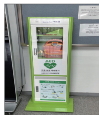
SolGeo Dormitory - AED
